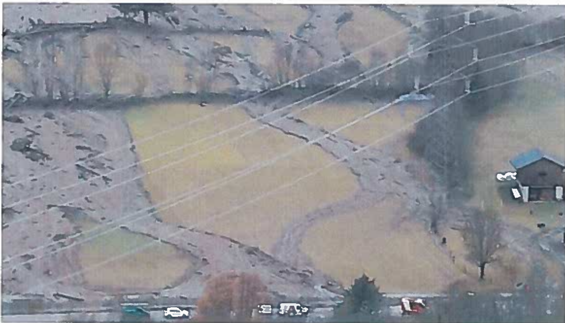
Photo 10: Landslide at Rangersdorf
