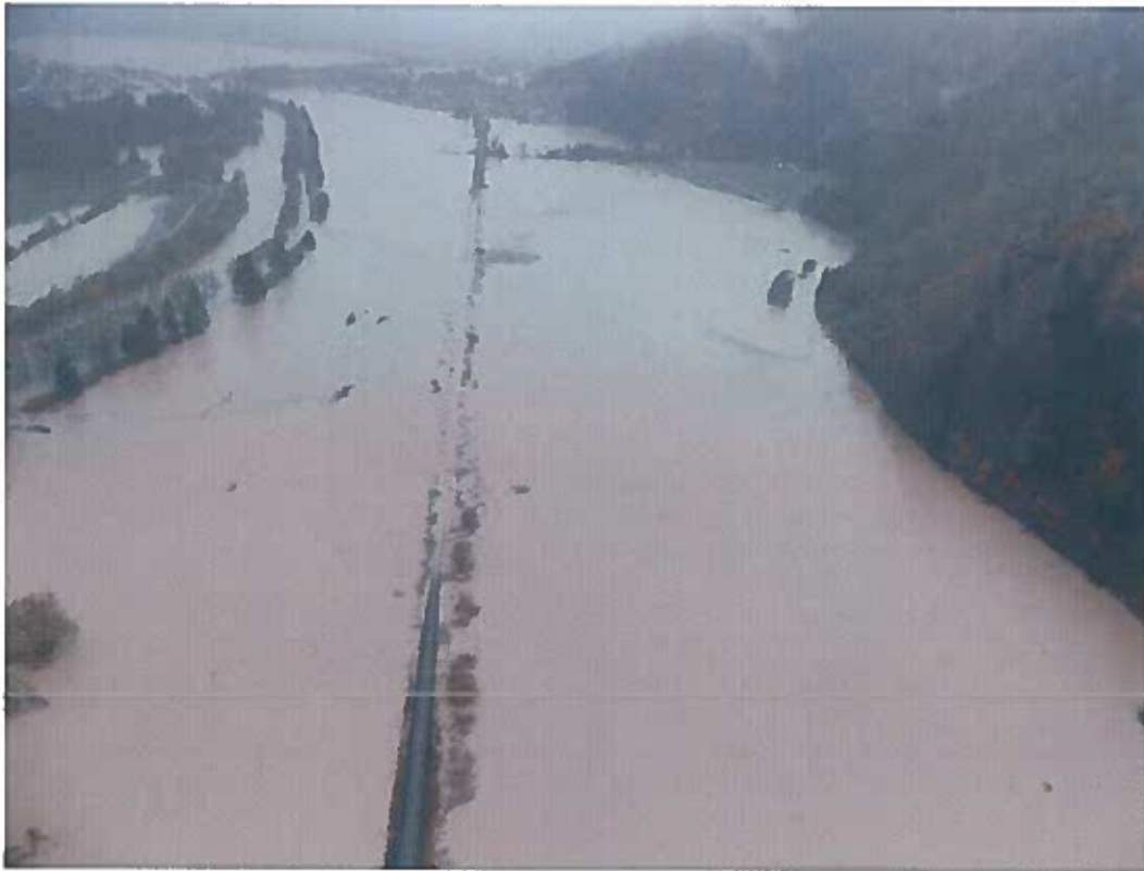
Photo 15: Gail at Tröpolach (old railway line)
